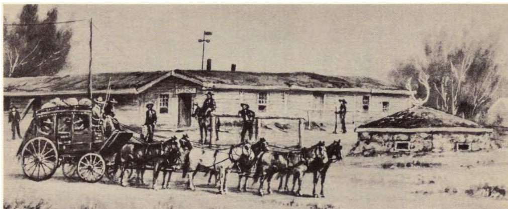
HAT CREEK STATION ON SAGE CREEK
