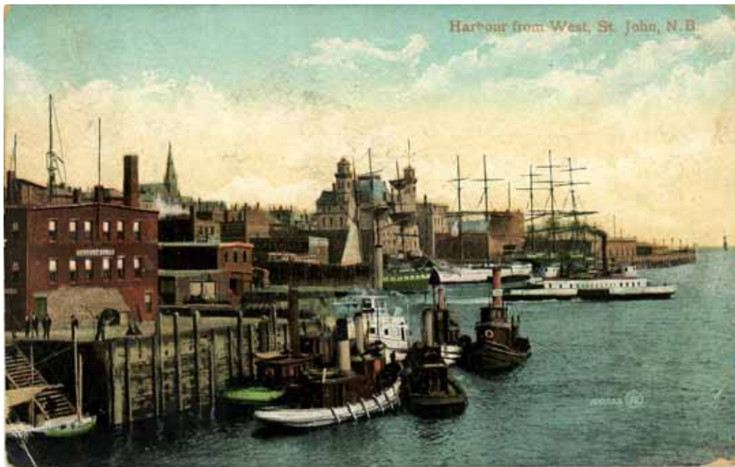
Harbour from west, Saint John
