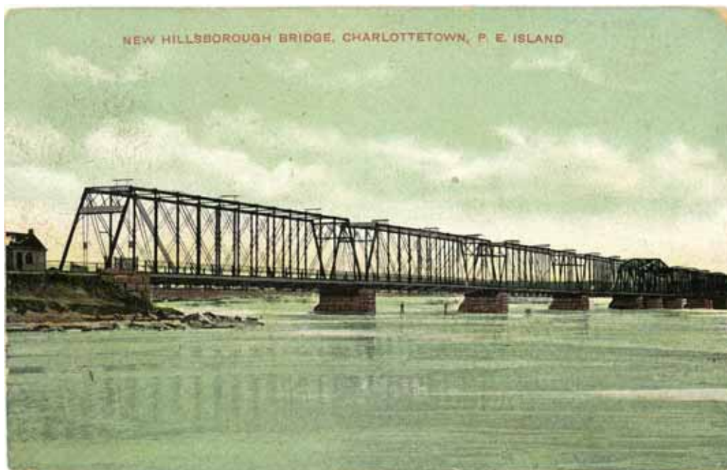
New Hillsborough Bridge, Charlottetown
