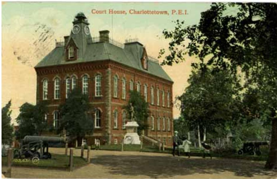
Court House, Charlottetown.
