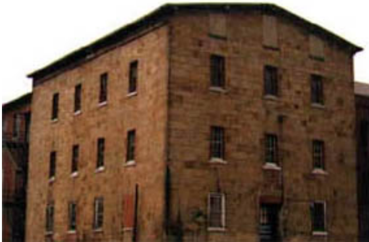
Photo of remaining portion of Jackson's Mill.
