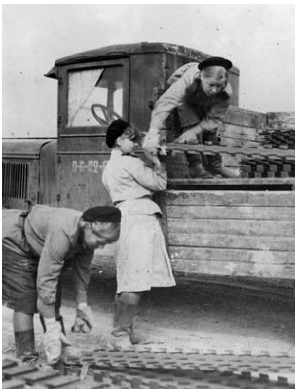
Red Army women assigned to Poltava in April and May 1944 laid steel mat for the runway that would accommodate American shuttle bombers.
