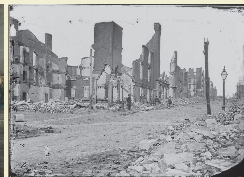
Ruins in the Richmond commercial district (Matthew Brady)
